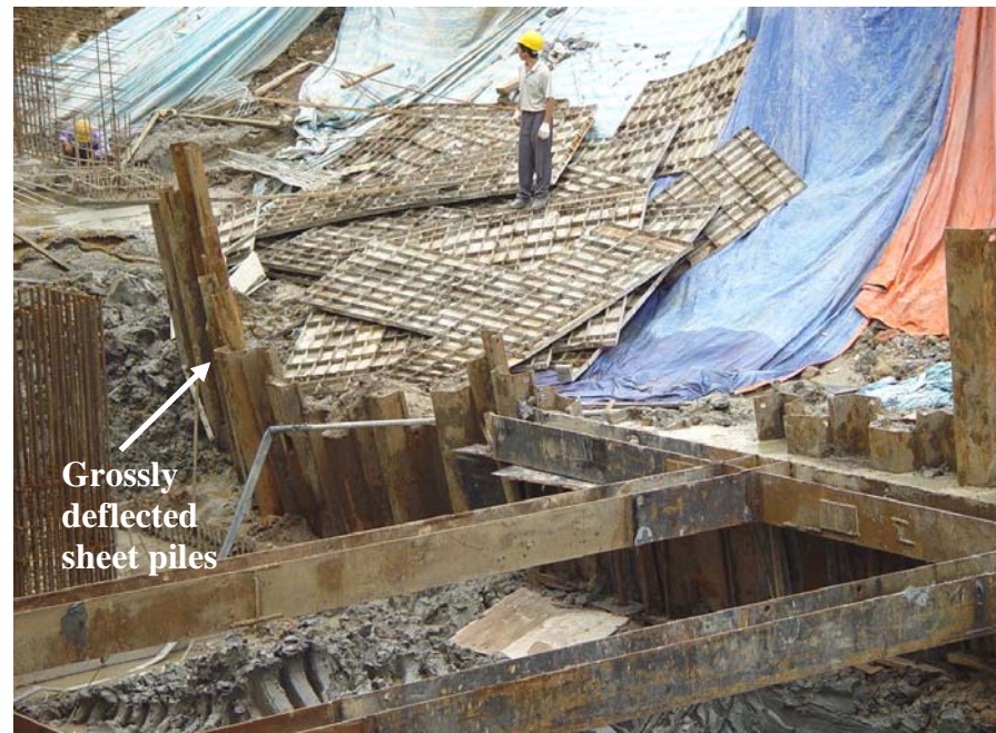
(g) Installation of struts when soil movement is uncontrollable (28 Dec 2002 – 2 Jan 2003)
