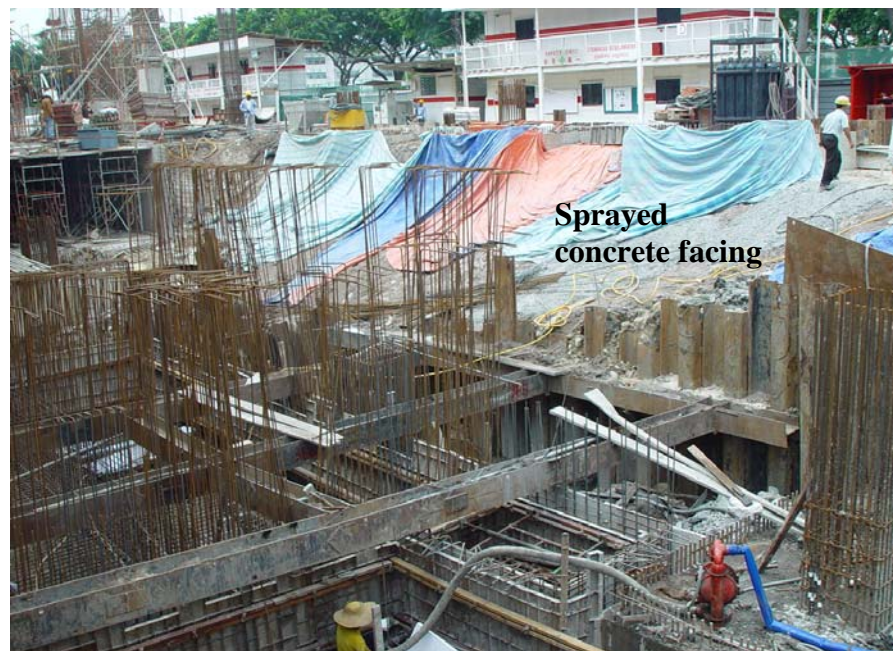
(h) Casting of pile caps for underground water storage tank (9 – 17 Jan 2003)
