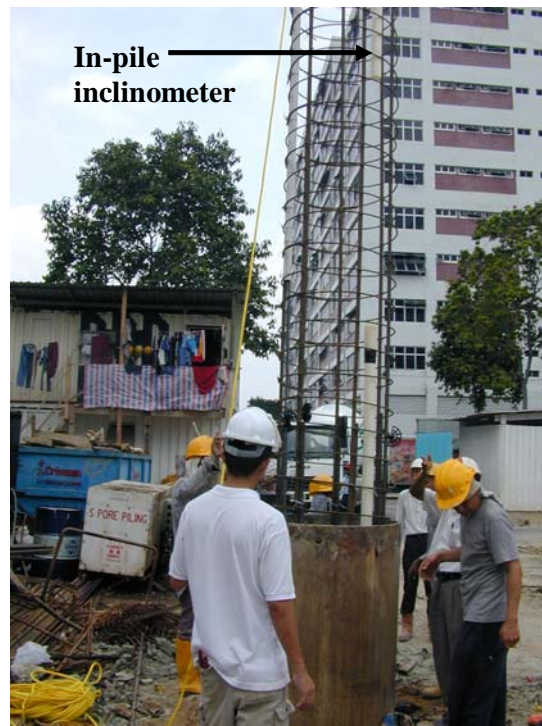
(a) Lowering of reinforcement cage into the ready-to-cast bored pile (5 Dec 2002)
