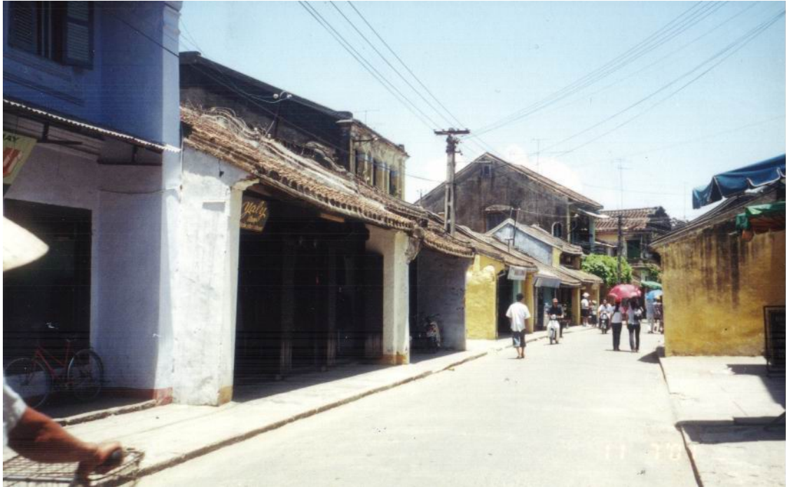
Picture 19: Unsightly electrical cables lining the skyline of Hoian.
