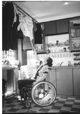
Figure A4.20: Hanging device was too high for wheelchair users to reach.
