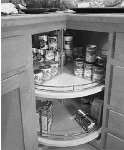
Figure A12.1: Rotating storage unit could increase the access to the interior of the cupboard at the corner (Source: Joliet Cabinet Company, 2003).
