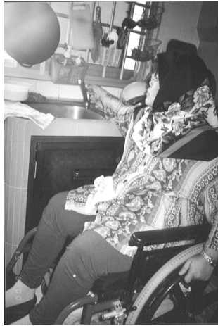
Figure A4.9: (Left) Ms. Nornilinda could not reach the handle of the faucet while sitting laterally at the sink.
