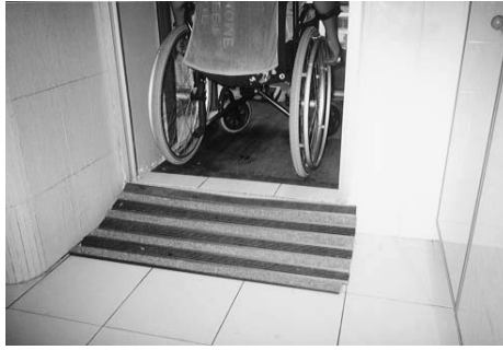
Figure A4.2: A simple ramp made for access.
