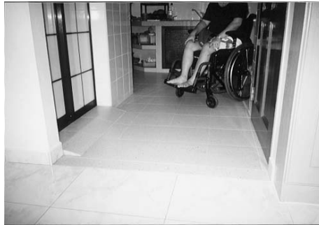
Figure A4.3: In Ms. Lin's kitchen the floor had been raised up to the level of the living room.
