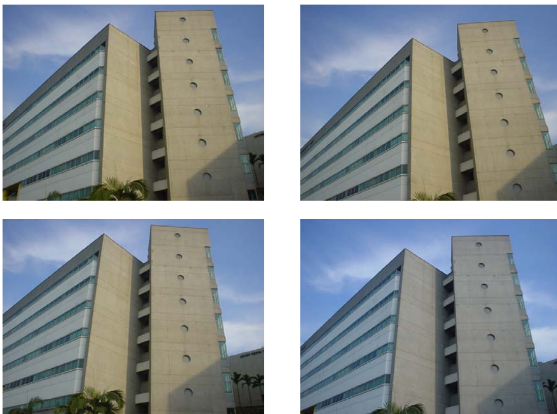
Figure 6.12: some images of a building
