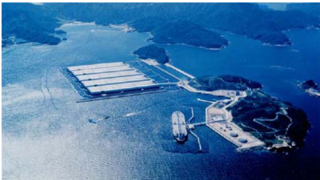
Fig. 1.2 Kamigoto oil storage base (Suzuki, 2005)
