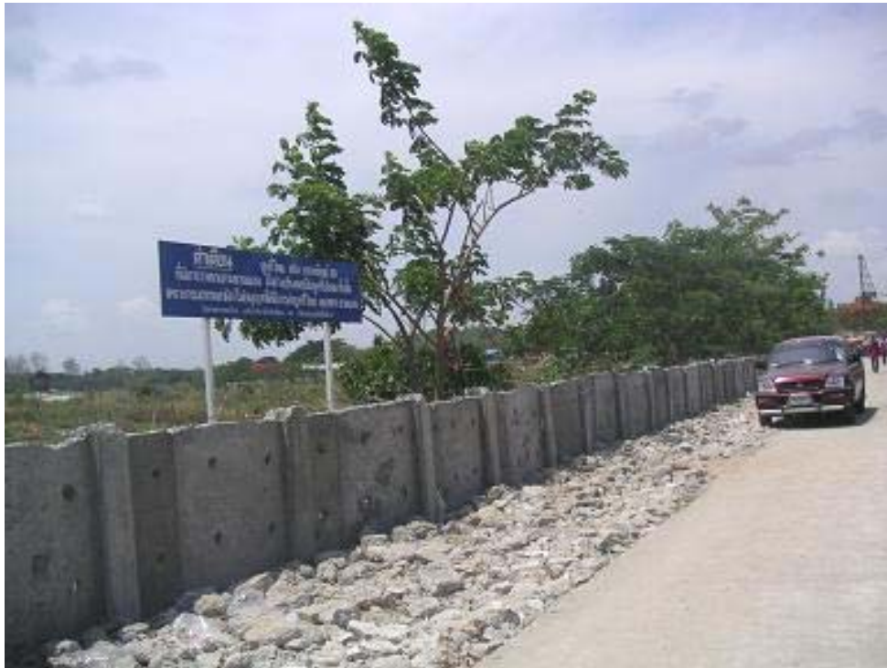
Plate 4.6 The Wall in the Building Process
