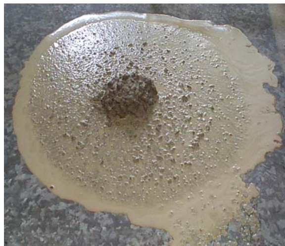
Fig 8.7: Observation of segregation by visual inspection
