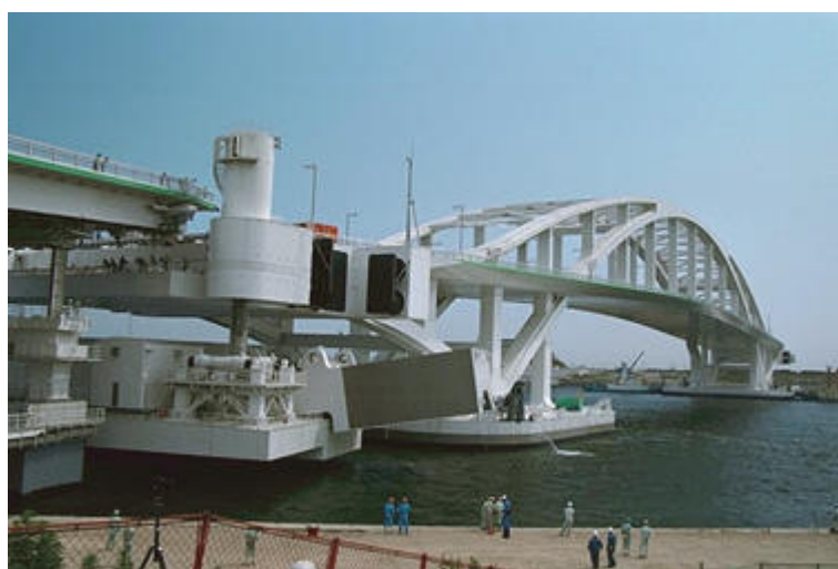
Fig. 1.3 Yumemai floating bridge
