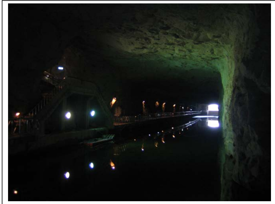
Plate 4.8 Zhaishan Underground Tunnel
