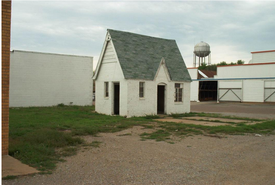
Figure 40. Cottage gas station. Altus, Oklahoma. National Park Service, Route 66 Division.
