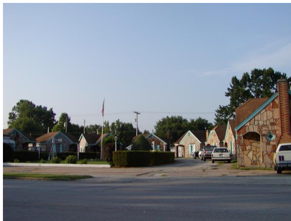
Figure 39. Cottage motor court motel. Springfield, Missouri. National Park Service, Route 66 Division.
