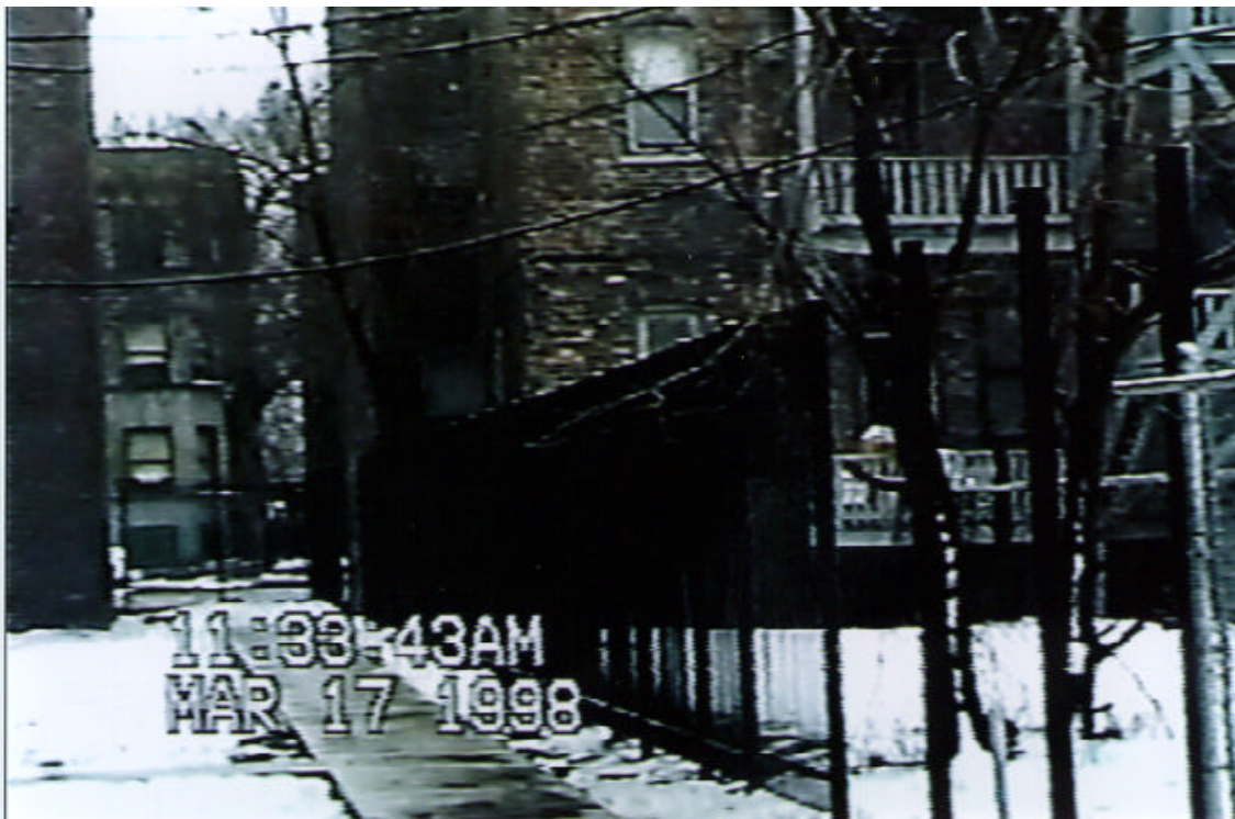
Figure 22. Wrought iron fence installed as part of the SECURE program .
