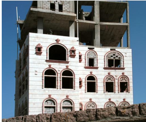
Fig 8. Al Habilayin. Mechanically cut stone making the façade of conventional concrete structures
