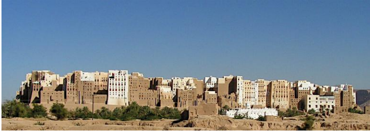
Fig 13. Shibam, chosen by the UNESCO and by the Aga Khan Award of Architecture as a model of what was and should be.
