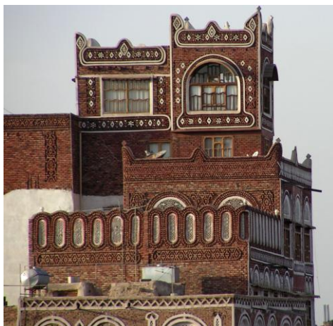
Fig 6. Sana'a. Baked brick as a means of flamboyance in the 21 st century. In the foreground, the roofline of an older and more subdued option
