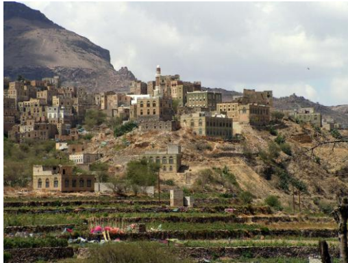
Fig1. Al Radma. Although contaminations from the 1970s on are evident, this settlement is representative of the prevalence of the architectural forms of the western mountains
