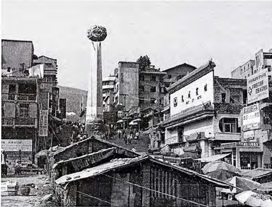
Photograph 3.1. The Ghost Head standing in Fengdu before 2003
