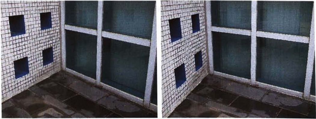
Figure 31: Image 1 and image 2 of the walls and ground of a building
