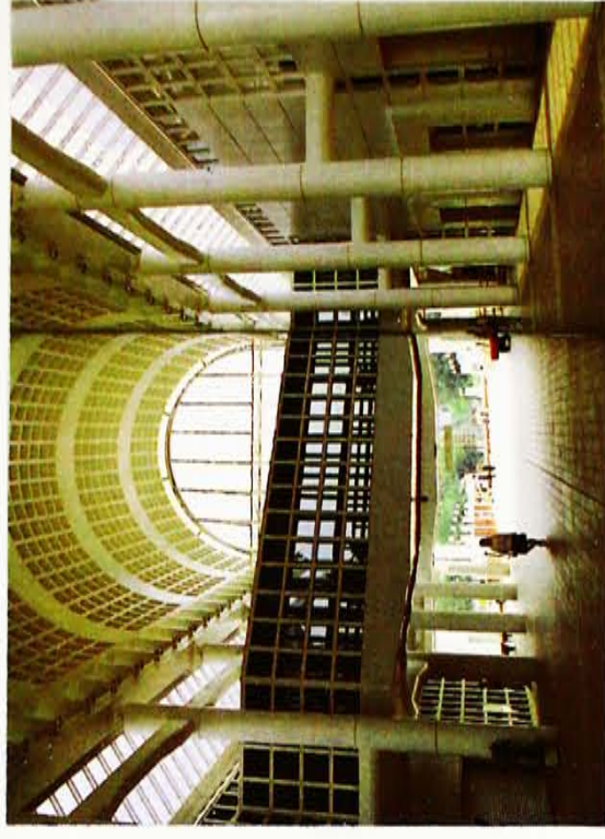
photo 4.3.2 The barrel -vaulted central concourse 20
