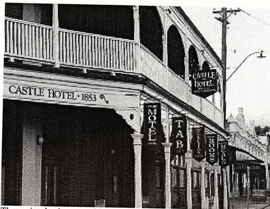
These simple signs provide all the necessary information to the customer and passer-by.
