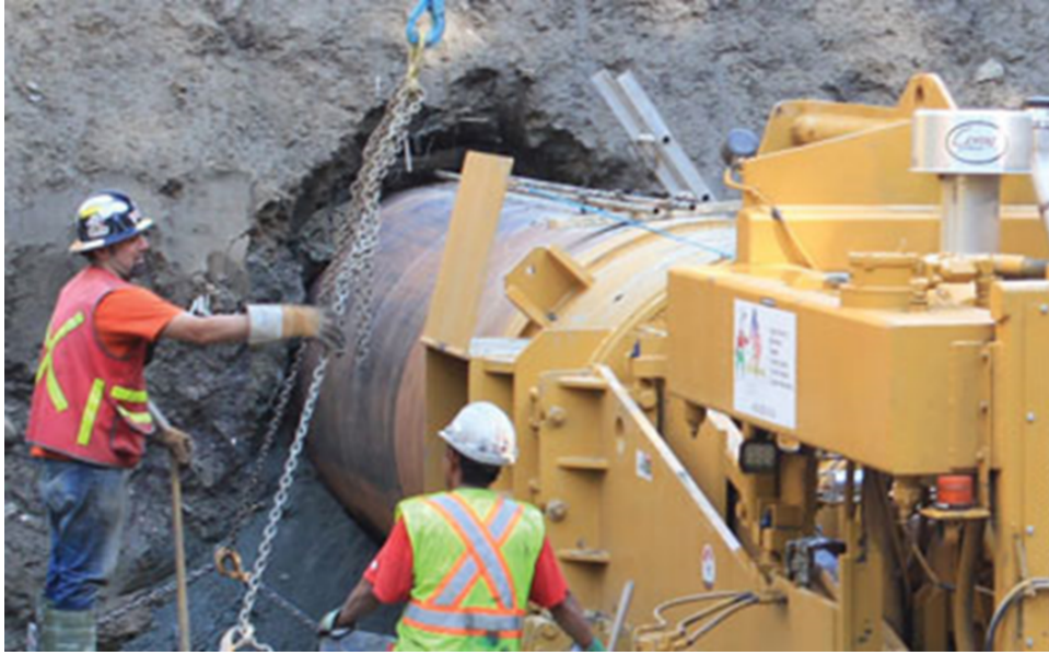
FIGURE 1.10 Pipe jacking (Side View). (Source: ISTT.)
