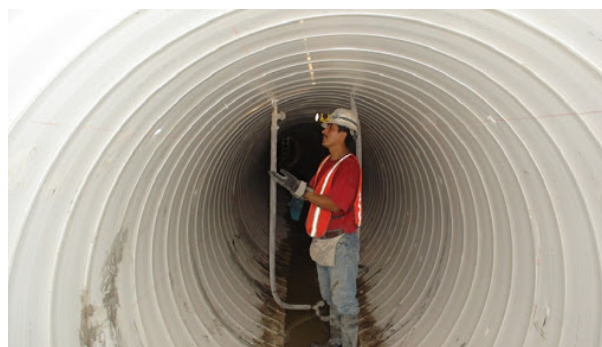
FIGURE 2.30 Internal feature of spiral winding. (Source: ISTT.)
