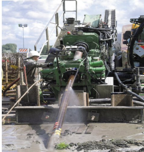
FIGURE 1.31 HDD Operator pullbacks drill rods. (Source: ISTT.)
