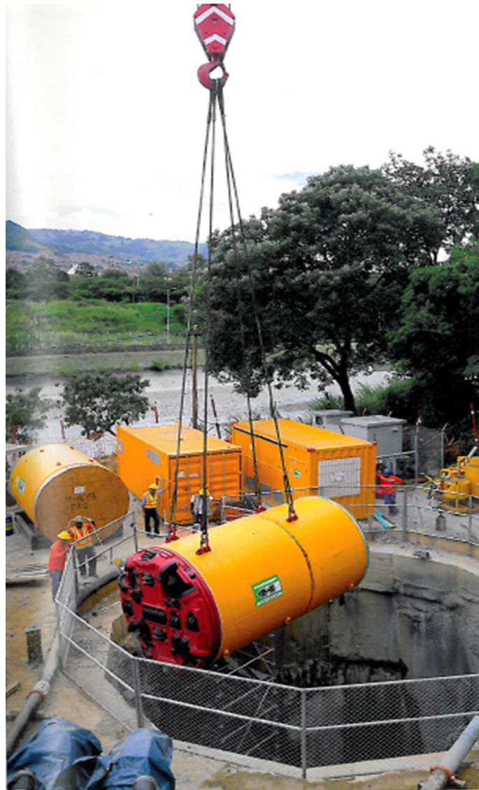
FIGURE 1.13 Pipe jacking microtunneling machine is lowered into shaft. (Source: ISTT, 2014)
