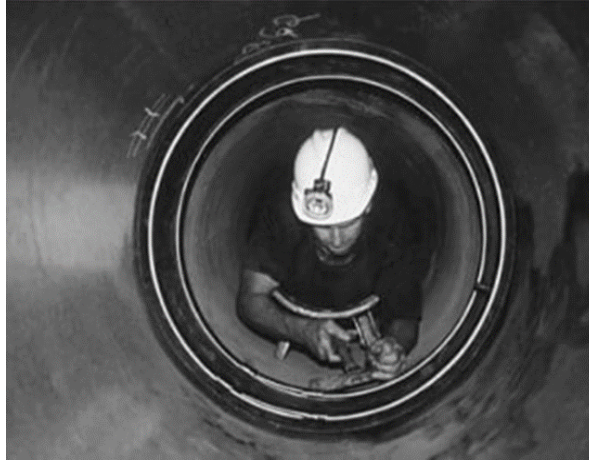
FIGURE 2.37 Localized repairs. (Source: ISTT.)
