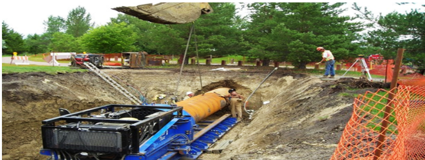
FIGURE 1.25 A construction work with horizontal auger boring. (Source: https://www.stantec.com/en/ideas/market/water/trenchless-technologies-horizontal-auger-boring )
