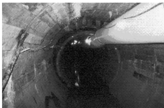
FIGURE 1.19 Inside view of a utility tunneling operations. (Source: ISTT.)
