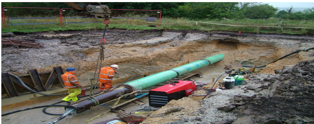
FIGURE 1.49 Pipe ramming machine in the field. (Source: ISTT.)
