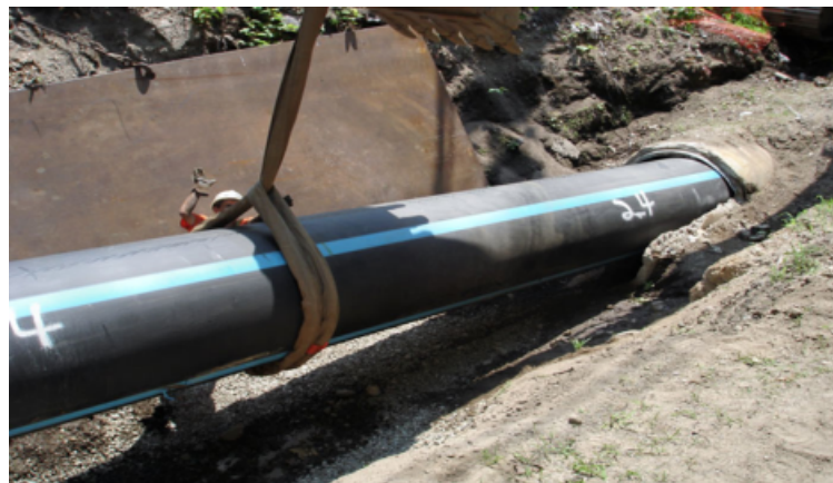
FIGURE 2.27 Sliplining. (Source: ISTT.)
