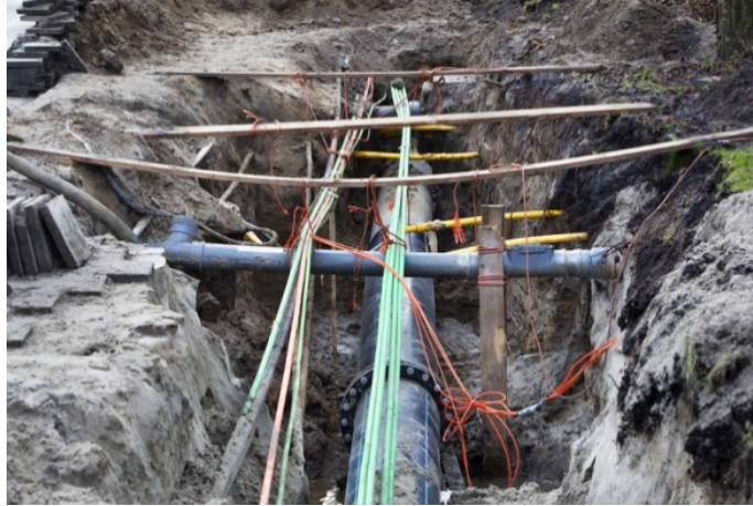
FIGURE 2.14 Underground pipe networks. (Source: www.plowmancraven.co.uk/services/gyroscopic-mapping-services/ )
