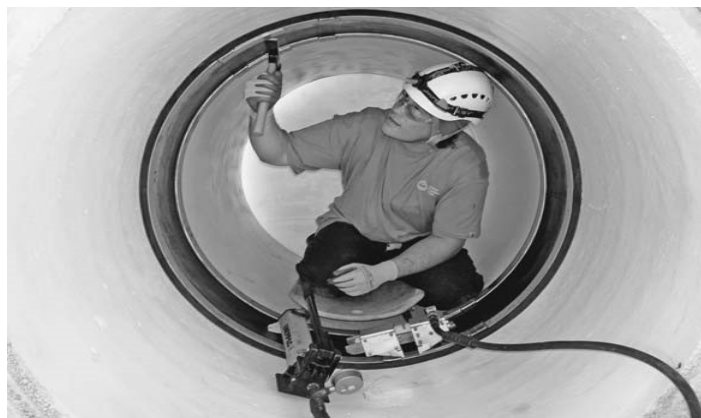
FIGURE 2.36 Internal seal point repair. (Source: Miller Pipeline Corporation.)
