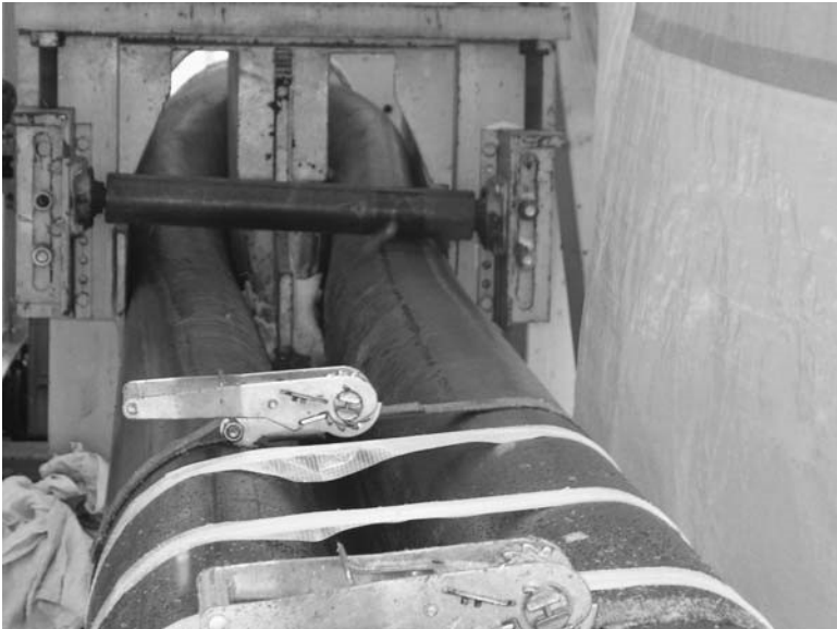
FIGURE 2.33 A semi-structural close-fit pipe going through diameter reduction process. (Najafi, 2010)
