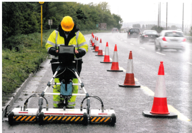
FIGURE 2.4 Mapping the underground by ground penetrating radar (GPR). (Source: ISTT.)
