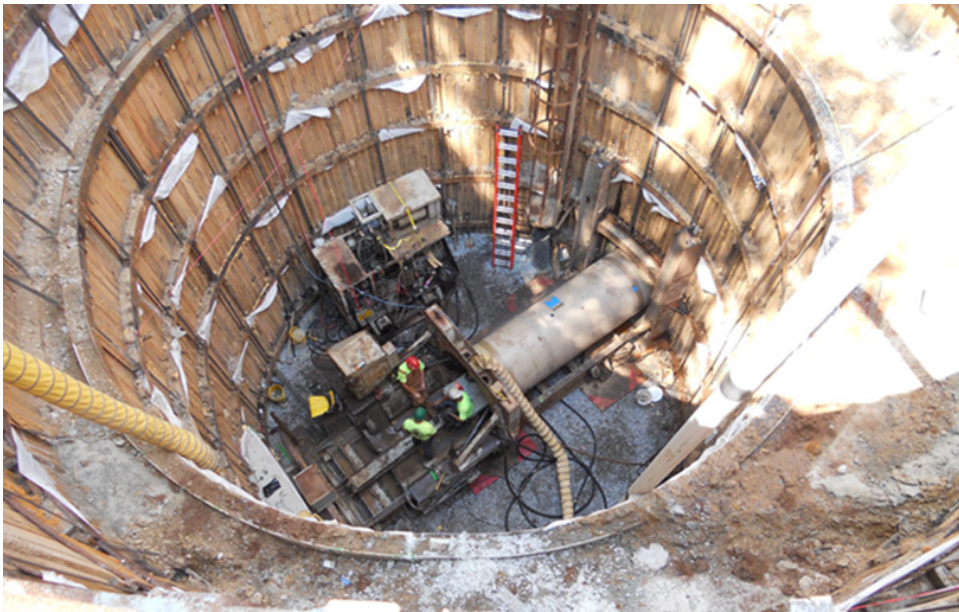
FIGURE 1.11 Pipe jacking (Top View). (Source: ISTT.)
