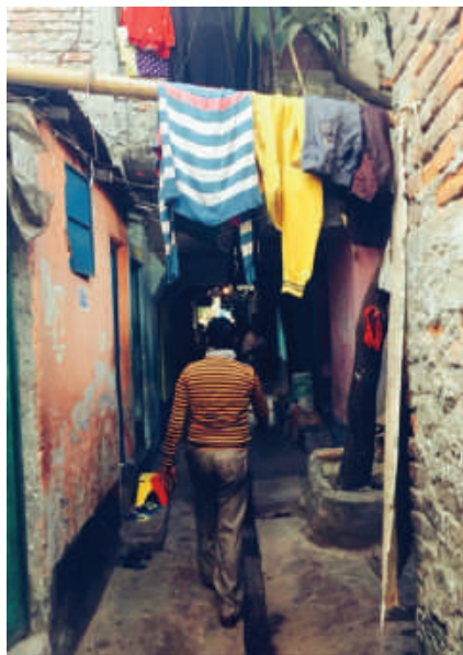
Figure 21: Surface drain in narrow pathway.
