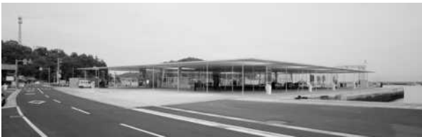
Figure 2. Ferry Terminal (2005) in Naoshima (Source: Márquez, F. and Levene, R., 2008, pp.104-105).
