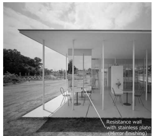
Figure 6. Resistant walls with the stainless steel plate reflecting surroundings (Source: Márquez, F. and Levene, R., 2005).
