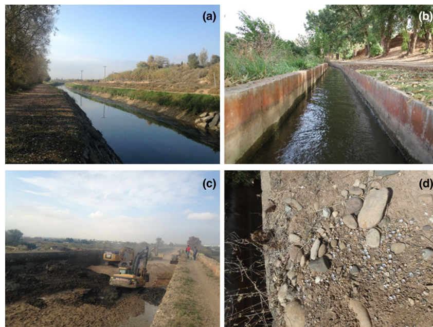
BOX FIGURE B1 Canal Imperial in Aragon (Spain) (a), Bouhlou Irrigation Canal (Morocco) (b), maintenance works in the Canal Imperial (c) and sediment and empty shells of several bivalve species after cleaning activities by farmers in the Bouhlou Irrigation Canal (d) [Colour figure can be viewed at wileyonlinelibrary.com ]
