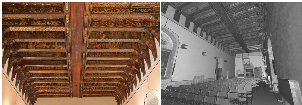
Fig. 1. Photo and a preview of a laser scan of the ceiling.
