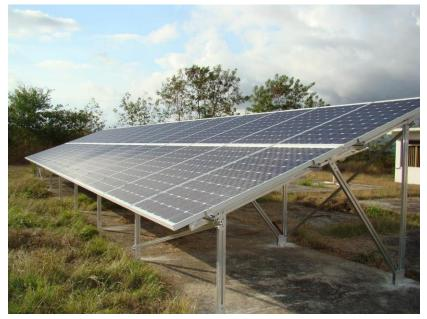
Figure 1. PV Microsystem 7.5 kWp
