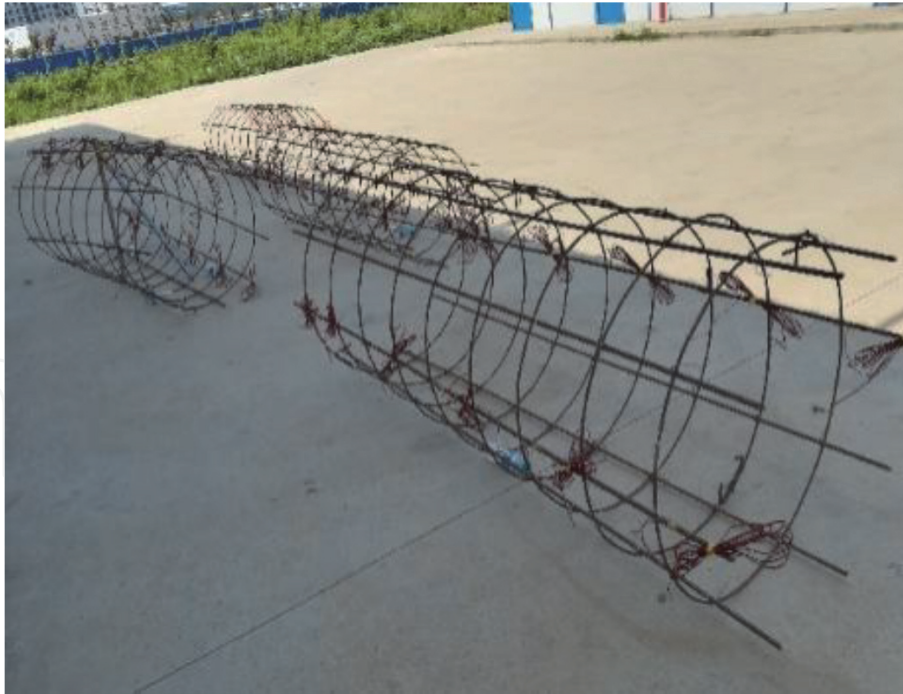
Figure 3. Steel reinforcement cage.
