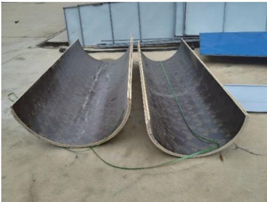
Figure 4. Molds for concrete casting.
