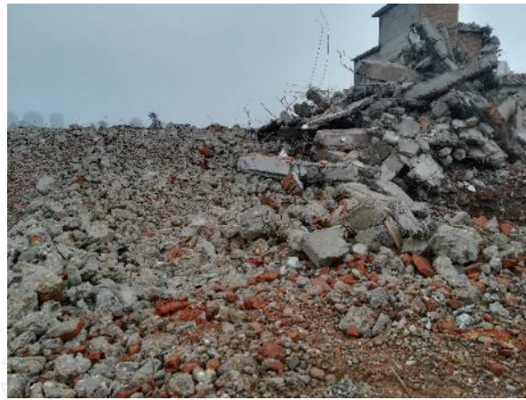
Figure 1. Demolition and transformation of DCLs.
