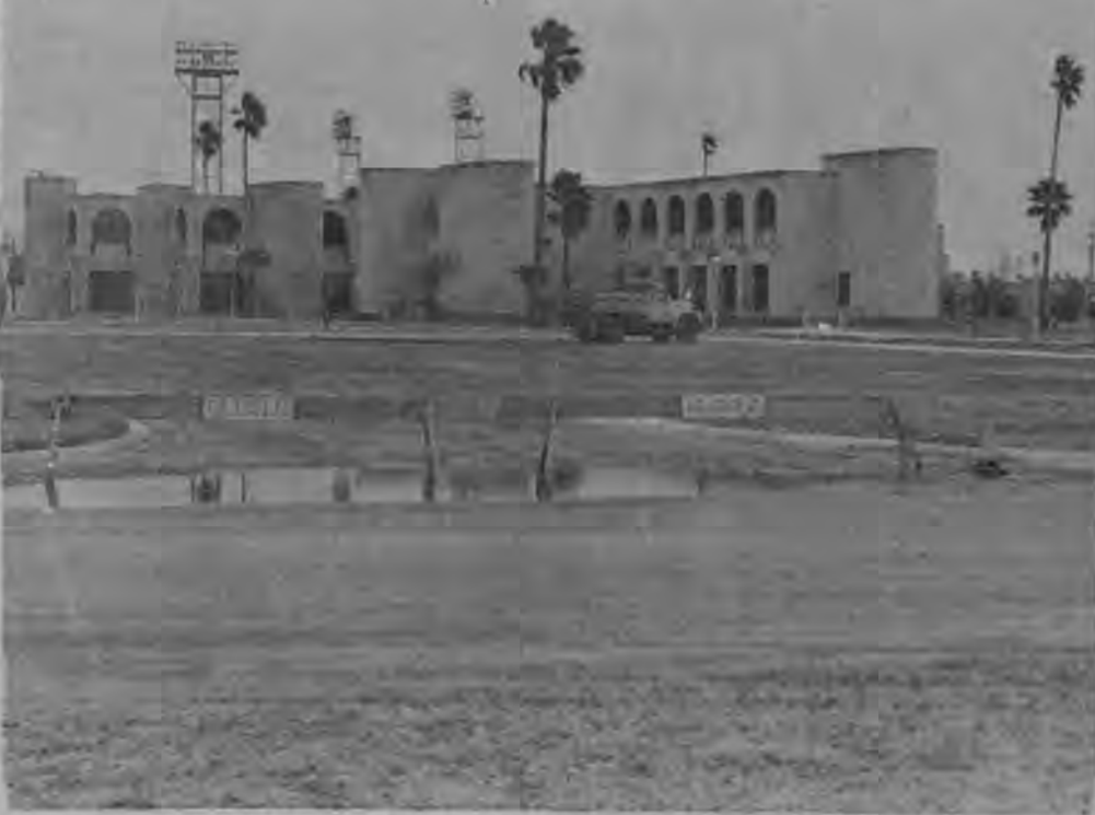
PARKING LOT NEAR COMPLETION —The site of the new parking lot to be completed in a couple of weeks is between the Education Building and the New Administration Building. The new lot will be reserved for faculty parking.
