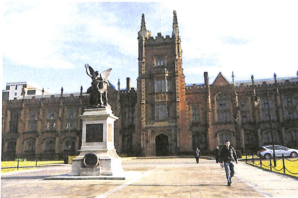
Figure 41. The great façade of the Lanyon Building at Queen's University Belfast; modeled after Gothic and Tudor medieval universities, this monumental structure “create[s] an instant authority and presence” (Stelfox, Latimer, & Evans 4). The colors of the red brick and sandstone are present throughout the city. 2010. Belfast. Photograph by author.
