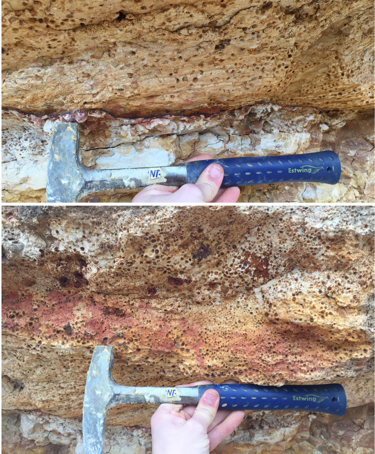
Figure 1.2. A photograph showing the contact between the interpreted friable fragmental unit and the lateritic duricrust.
