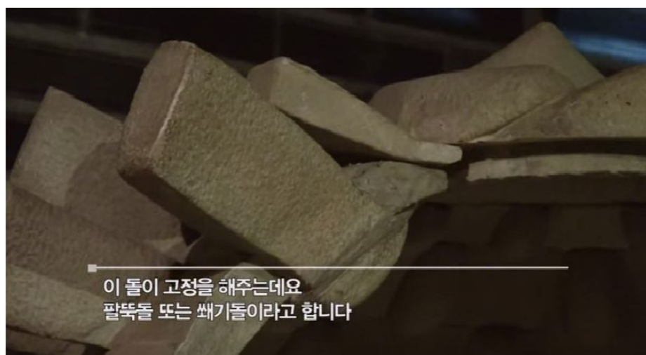
Figure 11. ‘Forearms’ that balance the horizontal and vertical forces at Seokguram’s cupola.
