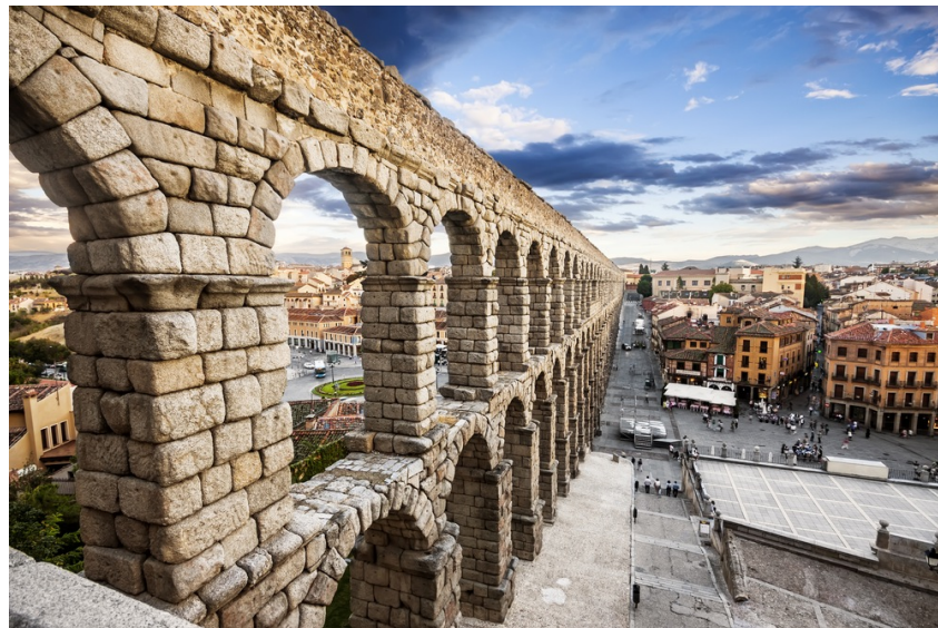
Figure 4. Aqueduct of Segovia (Spain). Granite ashlars without mortar.
