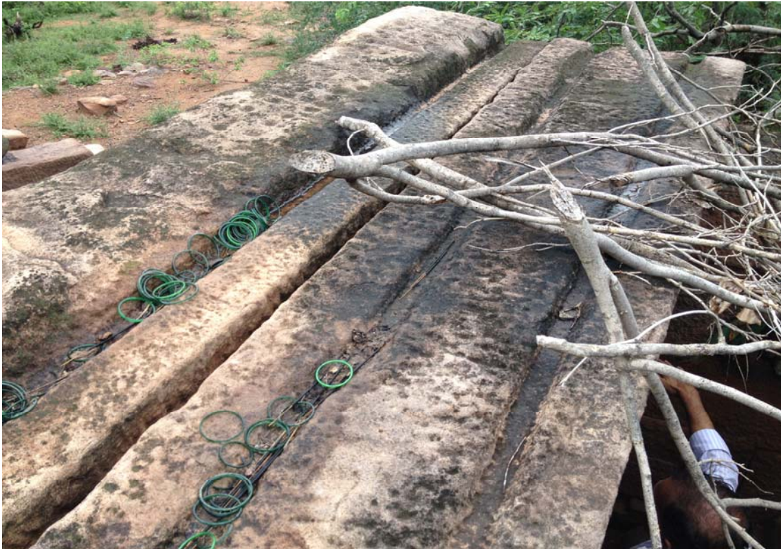
Figure 8: The roof of the shrine
