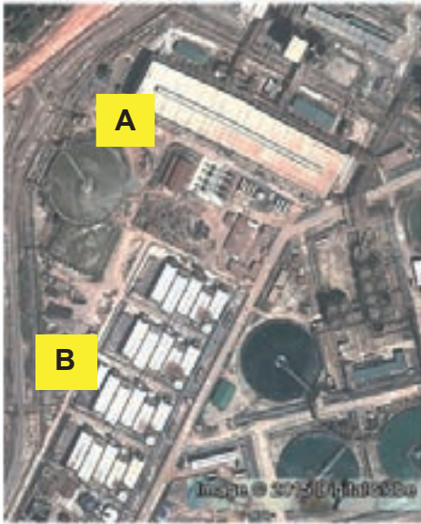
Figure 7: Google Earth image of Nchanga Copper mill (A – Electrowinning, B – SX)
