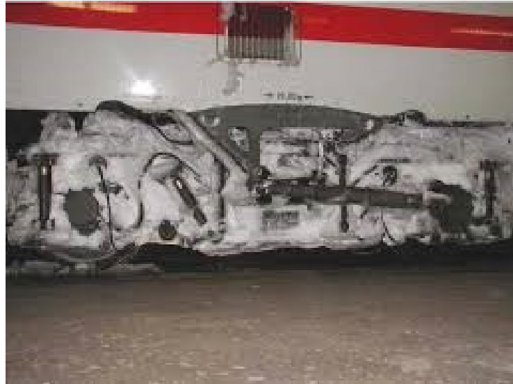
Figure 7. Snow packed on the underside of a train. [7]
