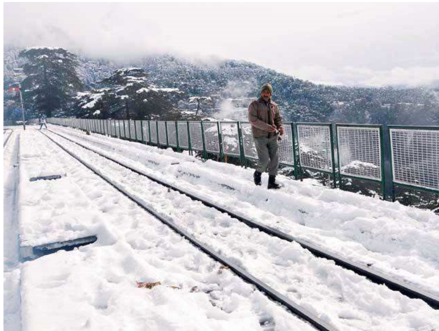
Figure 2. Railway tracks covered in snow. [20]
