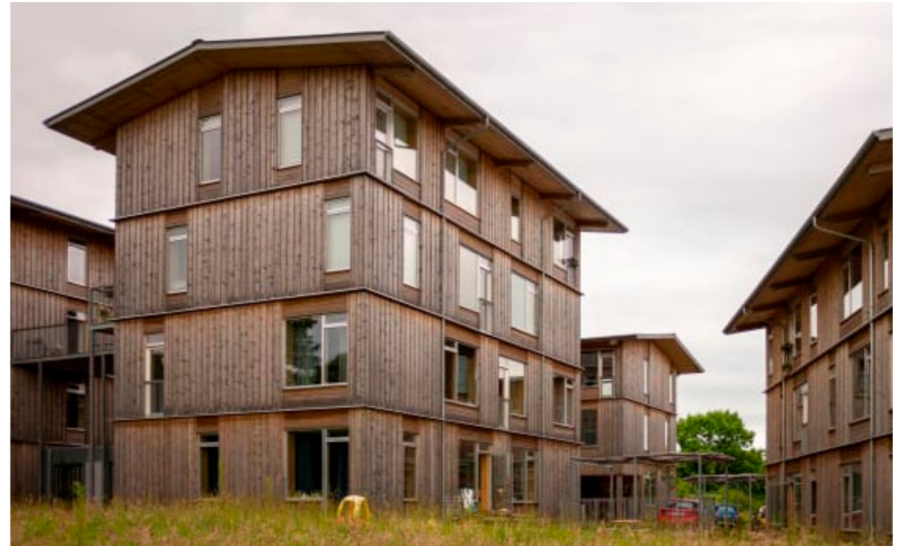
Figure 17. Wooden cladding is protected by overhangs and flashings, Lisbjerg hill, Vandkunsten (Mikkelsen 2021)
