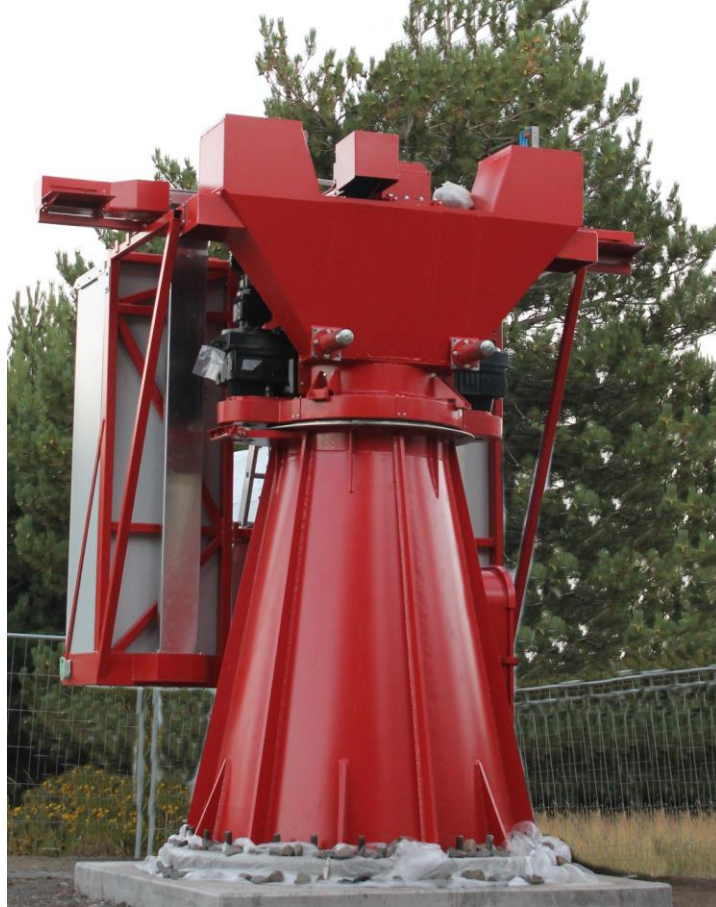
Figure 5: The mount structure of the ASTRI SST-2M during its assembly at the telescope site. On top of the base the azimuth fork is already installed together with the electrical cabinets.
