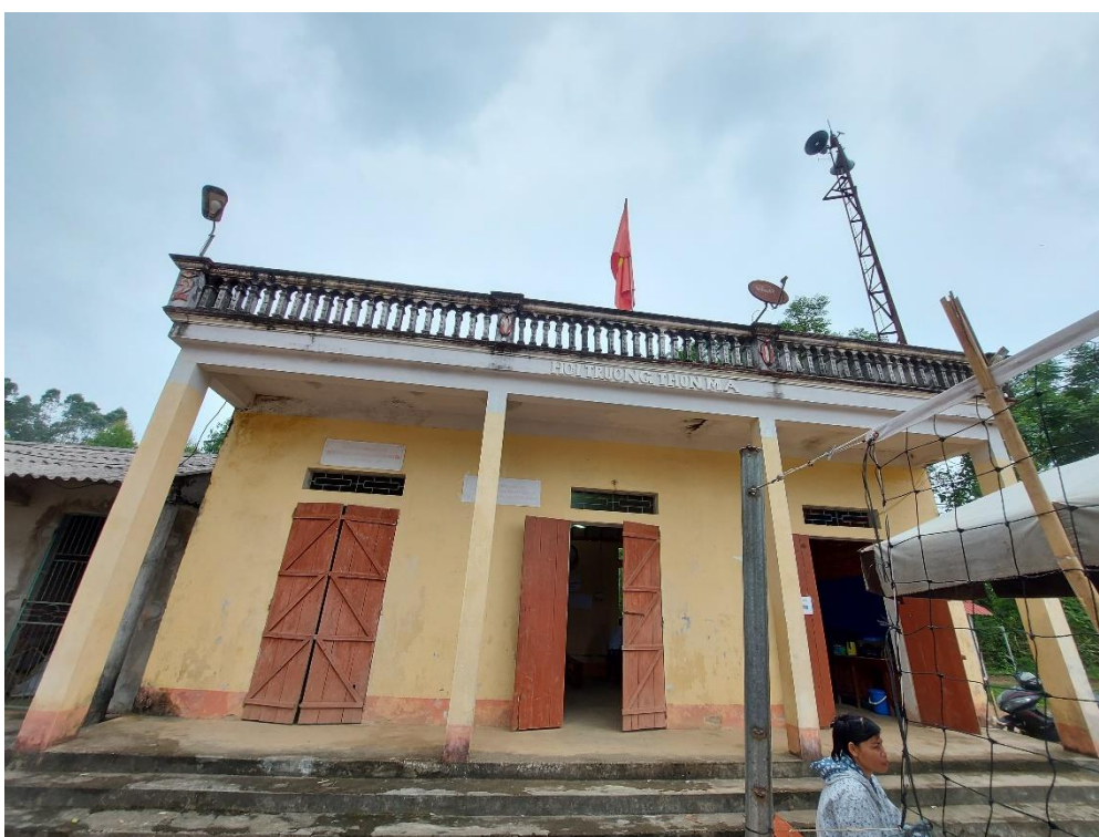
Picture 7. CSV's loudspeaker system in Vinh Kien
