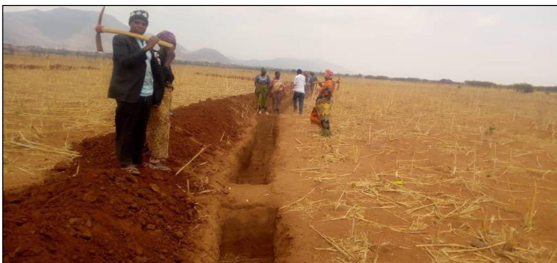
Figure 23. Farmers installing Fanya juu terraces in the field at Chemba district in Dodoma Region under Africa RISING/LEAD Foundation partnership in early September 2021. Photo credit: E.Y. Swai/TARI.
