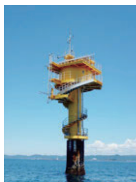
白浜海象観測所・観測塔 Shirahama, Tanabe-Nakashima observation tower
