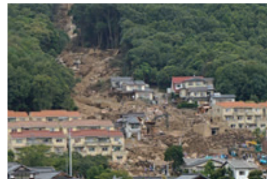
宅地への土石流の氾濫 (2014年広島) Inundation of debris flow to residential area (Hiroshima, 2014)
