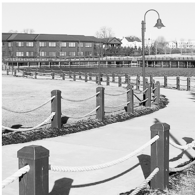
MBNA built the two-story call center in 2001 and developed the 10-acre waterfront property, including a popular open-to-the-public walkway. About 300 people worked at the center when it closed in 2005. Bank of America acquired the property when it bought MBNA in 2005.
