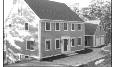
New dream home by local master-builder must be seen to be appreciated: 4,000 square feet of heated area includes the finest and most luxurious living imaginable, all on a beautiful wooded Rockport lot convenient to everything. Professional landscaping is icing on the cake. $720,000
