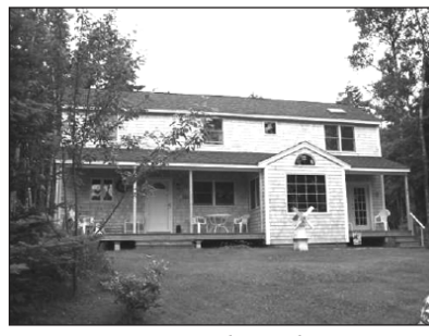
Otis Point, St. George: Fine home with 33' ROW - nice beach and deep water access. Cedar shingles, Andersen 400s windows, 2 farmer porches with Timber Tech decks. Two rooms still need to be finished inside. Sailor's paradise on mile-wide river. $299,900
