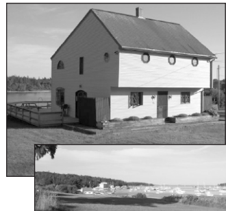
Views from all rooms in this Tenants Harbor Village home. Wonderful Garrison Colonial style home within a stone's throw of the water. ROW comes with this treasure. Large formal rooms, finished with care, quality construction. $739,000
