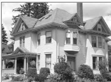
1896 Queen Ann Victorian-Free Classic Style, Rockland: Meticulously restored 6-BR/3.5-BA home with grand foyer, oak floors, custom oak kitchen, 3rd floor nanny's quarters with separate utilities. 3,503 sq. ft. finished living area. Excellent location. $449,000
