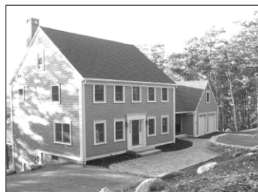
New dream home by local master-builder must be seen to be appreciated. 4,000 square feet of heated area includes the finest and most luxurious living imaginable, all on a beautiful wooded Rockport lot convenient to everything. Professional landscaping is icing on the cake. $750,000
