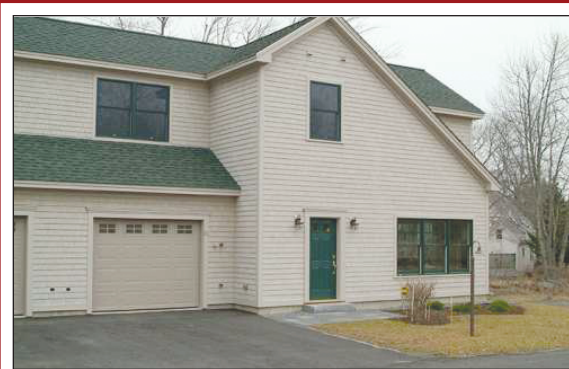
CAMDEN: New condominium complex, Wiltshire Place, has seven units planned. Unit #1 has 4 BR, 3.5 baths, hardwood floors, granite countertops, in-floor radiant heat, screened porch and attached garage. Enjoy one-level living with 1 BR on first floor. Walk to town. #788237 $399,000 Pat Jones 236-4777 PatJones@tcreal.com
