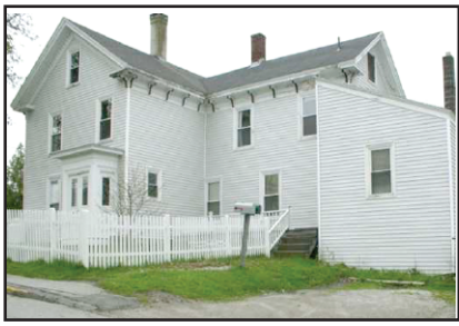
Only steps away from the boardwalk, this duplex has a corner lot and harbor views. Let your tenant help pay the mortgage! Watch the boats in the harbor from your deck! Rockland $250,000
