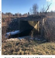
Corey Road (box culvert / fish passage)
