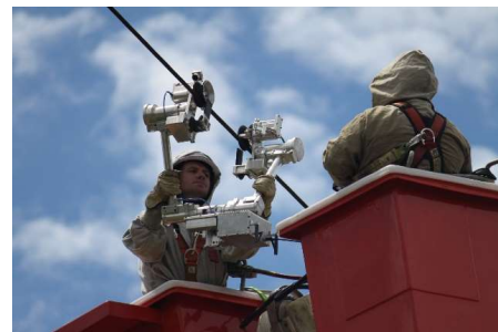
Figure 33 Manual, live-line placement on 80 kV line from a bucket truck.
