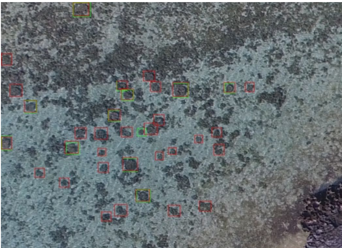
Figure 3.7: One detection example of group G5. The green bounding boxes indicate the ground truths while the red ones are the detection results.
