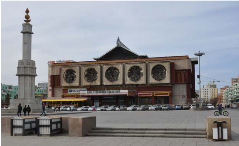
Figure 6: The Lenin Museum, Ulaanbaatar, G. Luvsandorj (design 1970s). Source: Photo by Łukasz Stanek, 2018.
