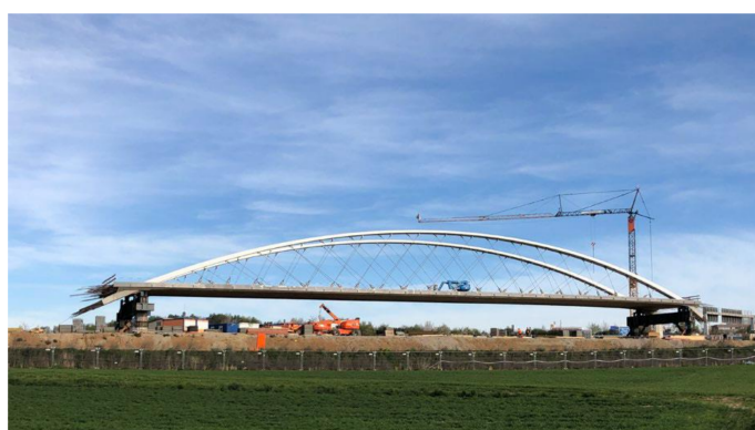
Figure 1. Network arch bridge with inclined CFRP cables [9], reproduced with permission by Prof. Urs Meier.
