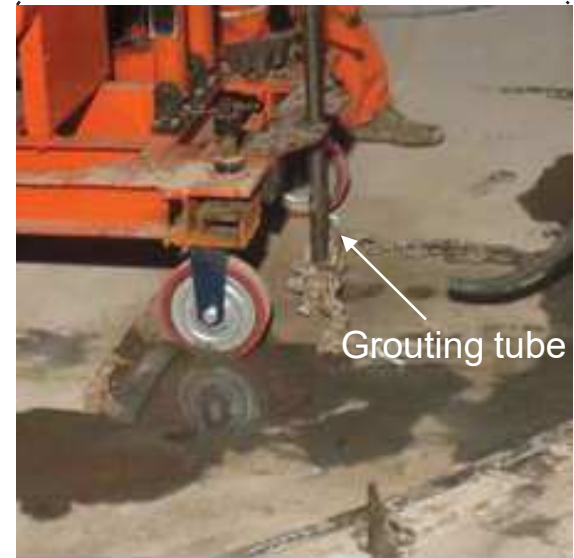
Grouting operation at the site
