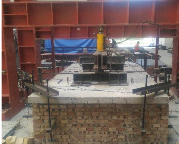
(a) Photograph of the test setup
