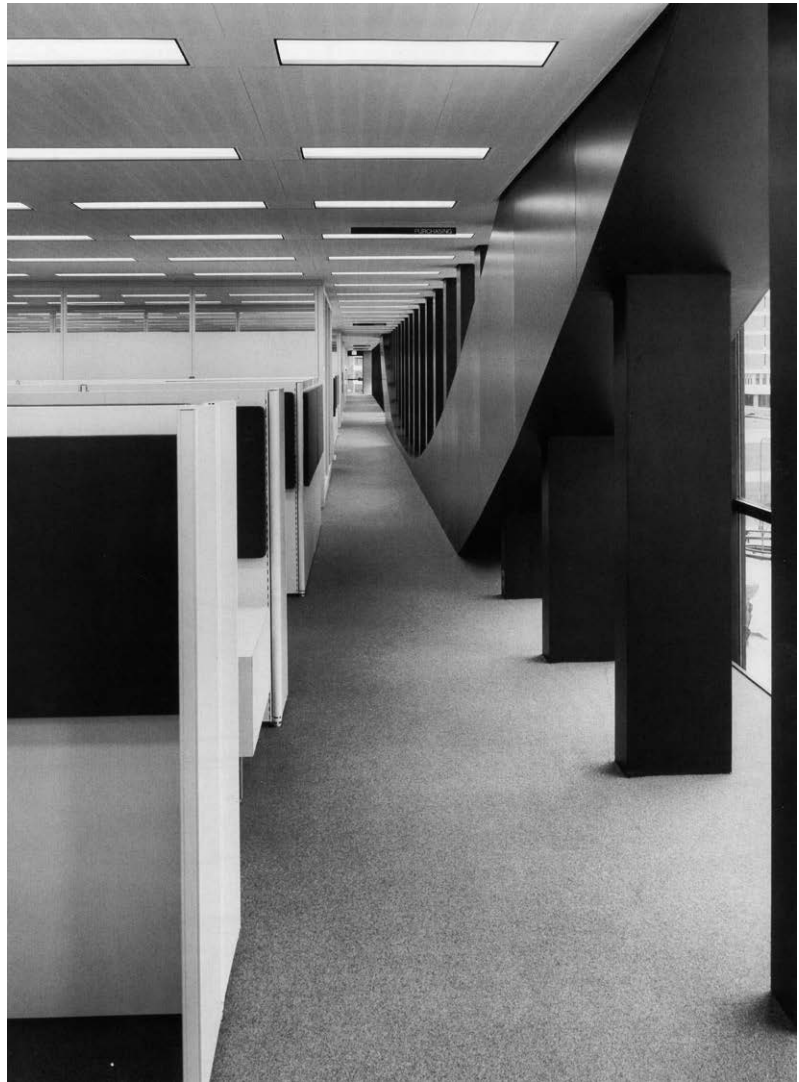
Fig. 10 Interior of the purchasing department on floor 2, the FRBM office tower, with workstations and demountable partitions by General Fireproofing at left, and the bottom of the catenary suspension structure at right. Photograph by Balthazar Korab, courtesy Library of Congress, Prints & Photographs Division, Balthazar Korab Collection.
